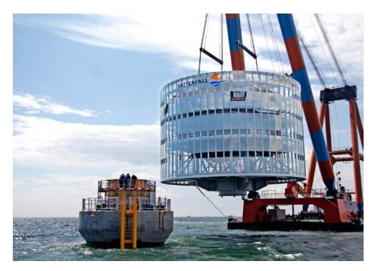
Picture 5. Installation of transformer station at Lillgrund (Photo: Hans Blomberg/Vattenfall).
